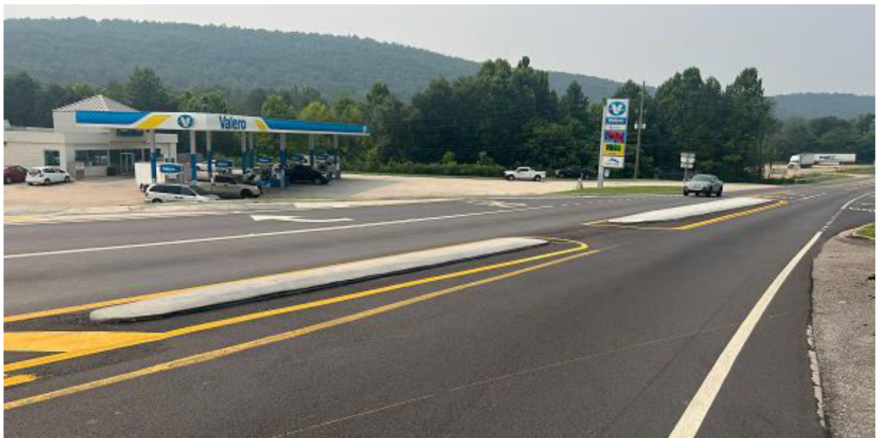
Photo 3: Kelly Creek Road improvements just south of I-20 eastbound ramps
