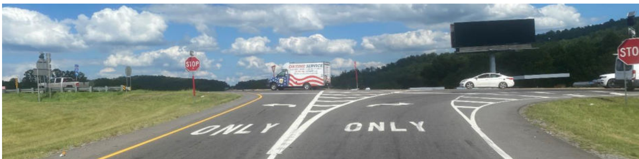
Photo 4: All-Way Stop-Control Condition at I-20 Eastbound Exit Ramp Approach to Kelly Creek Road
